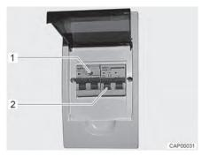
Fig. 90 230 V fuse box with safety cut-out and FI-switch
