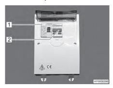
Fig. 116 230 V fuse box with safety cut-out and FI-switch
