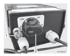
Fig. 126 Regulator for electrical floor warming unit
